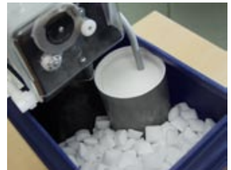
Plant seen from above without cover. Regeneration is adjusted on the front panel. Salt shall be filled in the salt tank in the middle of the cabinet. The plastic cabinet is set on wheels which makes cleaning underneath the plant easier. Note the simple installation.
